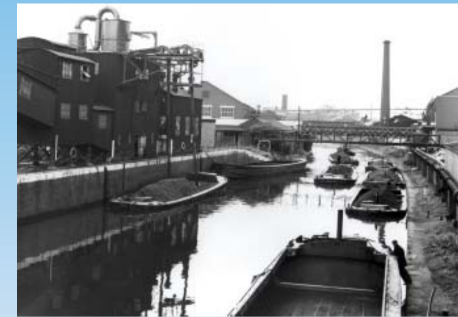
Barges unloading coal at Trafford Power Station.
