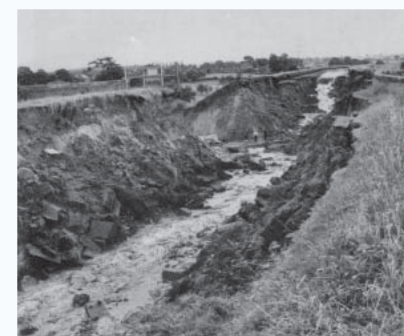
The 1971 breach of the Bollin aqueduct. Some idea of the scale of the collapse can be gained from the people in the centre of the photograph.
