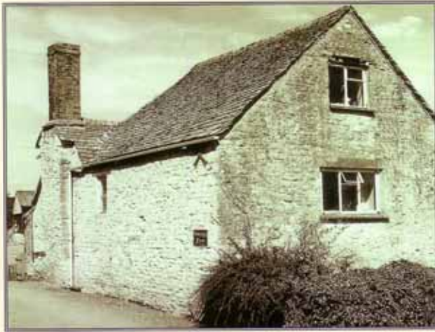
Oakridge Farm. The 1950's metal windows disguise the ancient origins of the farmhouse. This wing contains the walls and part of the roof of a small open medieval hall, dating to the late 15th century.
