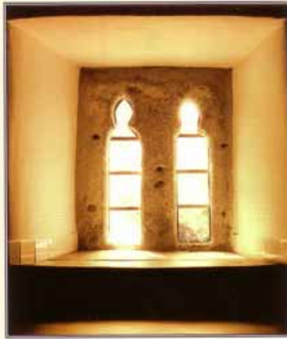
Medieval windows at Frampton Place.
