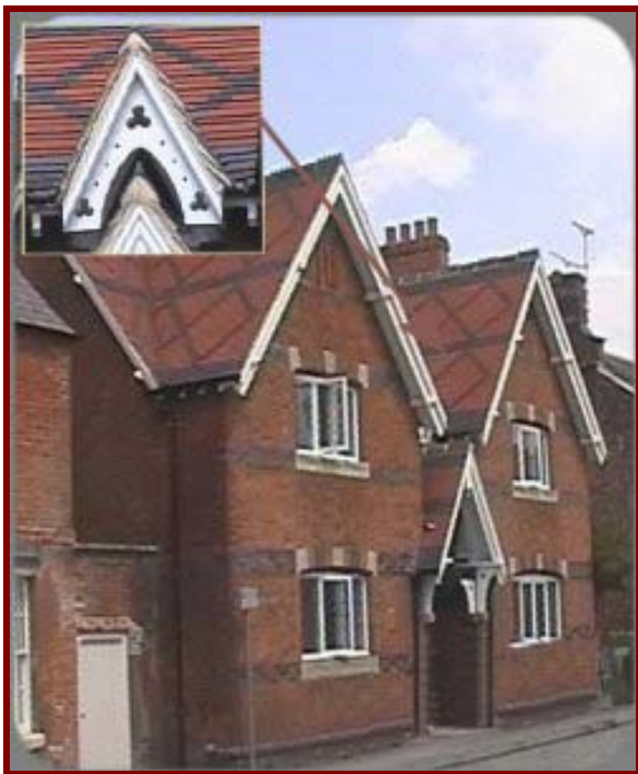
Chantry House, showing roof details
