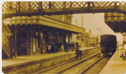
Above: Haverhill Railway Station
