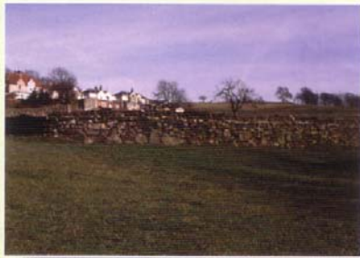
Where a wall is built over large stones it is very old
